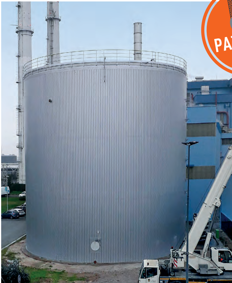
LIPP Gross-Pufferspeicher, 5.200 m 3 Volumen
